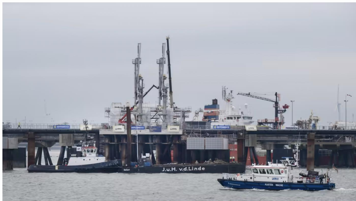
The new LNG terminal in Wilhelmshaven, Germany © David Hecker/Getty Images
